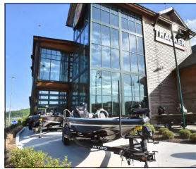
Bass Pro Shops, in WestRidge, has completed an addition facing I-79.
